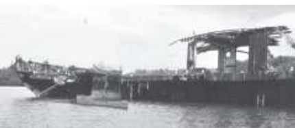
Remains of Mortlake Bank in 2003 near the western shoreline of Homebush Bay
