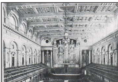
Sydney Town Hall: Wunderlich made the pressed metal ceiling.
